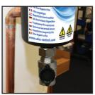
2 Close drain valve using drain cap, ensure the cap is alligned correctly so the valve is fully closed.
