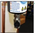
**6** Close drain valve using drain cap, ensure the cap is alligned correctly so the valve is fully closed.
