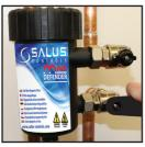
Important – Before carrying out any servicing work, turn off electrical supply to the boiler and let the water cool down to a safe working temperature. Using the Mag Defender spanner provided turn both isolation valves to the OFF position.
