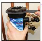
8 Now replace the lid onto the canister and tighten with the Mag Defender spanner. (Do not over tighten).
