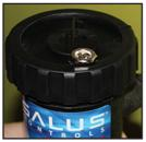
Bleed through top air vent, bleed the MD22A again after the system has reached temperature. Take care as the water will be hot.
