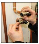
2 Now Loosen off the valve flange nuts and insert the rubber washers provided. (There are 2 supplied with this product).
