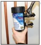
Grip the Mag Defender and tighten the compression fittings being careful not to over tighten as this may cause damage.
