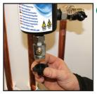
8 Replace cap on drain valve and run the central heating system. Bleed air through air vent if required.
