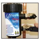
10 Open the isolation valves and start the heating system.
