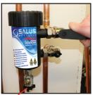
Now the heating system is ready to be filled, ensure the inlet and outlet valves are both in the open position, with the drain valve in the closed position, and then run the central heating system.
