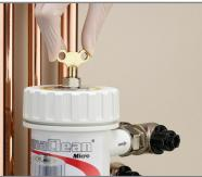
Open the isolation valves to the marked ON position and vent/bleed through the Pro-Fill air vent. Protect the surface below the canister with a dust sheet or container to capture any drops of water. Run the central heating system while checking for leaks. Repeat steps 1 - 6 if required. Ensure the filter is thoroughly clean before leaving the premises.
