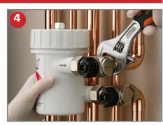
Loosely secure the MagnaClean Micro canister to the valves, following the flow direction indicated on the canister. Grip the canister and tighten the compression fittings being careful not to over tighten.
