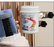
Unlock the bayonet screw on the base of the sheath and remove the debris collector. Rinse until all the non magnetic debris has been removed. Replace and lock the bayonet screw onto the sheath and place the sheath into the canister. Insert the magnet lid assembly and tighten until sealed.
