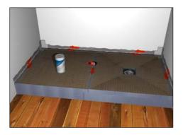
Where the shower area meets the wall apply a thin layer of tape sealer to the shower area and the adjoining wall approximately 60mm wide on both. Apply a thin layer of tape sealer across the joint between the shower tray and the shower tray extension to a width of approximately 120mm. If the shower area is not wall to wall and is having a glass side panel you only need one waterproofing internal corner not two.
