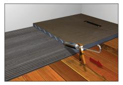
Open the Fix-MD adhesive tube and squeeze a wavy line of adhesive along the edge of the shower tray that will join with the shower tray extension using a sealant gun.
